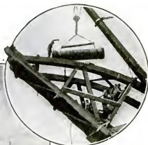
At the upper end of the cradle (above) pipe sections were laid one by one and joined. Then, as the barges supporting the cradle moved forward, the jointed pipe slid down a curved skid to a trench at the river bottom, as shown at left
