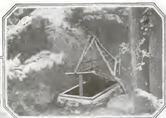
The water from the well above is automatically pumped to two farms. The pump is enclosed in the house to the left. When any faucet is turned on the water works against the piston of the pump
