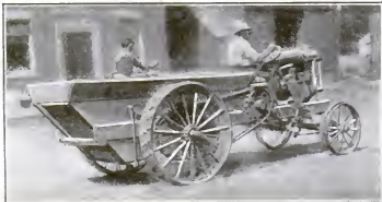
How Fordson tractor was combined with steam tractor wheels
