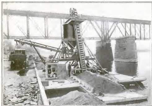
The flat coal-boat is slid in between two floats having a chain-and-bucket elevator; the coal is carried to a storage bin above and fed to a belt conveyer running to shore
