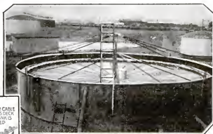
An oil tank made fireproof and evaporation proof by a newly invented roof that floats on the surface of the oil, thus excluding oxygen necessary for combustion
