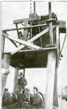
From a machine gun mounted on the top platform of this tower, bullets were fired straight upward. Half-inch armor plate covering the lower platform protected observers from returning missiles
