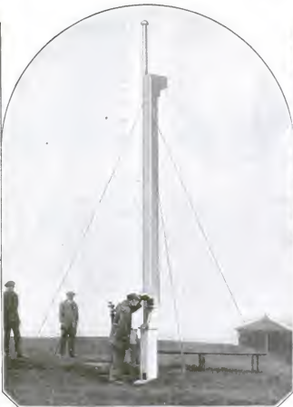
At a "blind" hole, the periscope is now solving a difficult problem for the golfer who can't see the flag on the next green. By peering into this 20-foot tube, he can find out whether "all's clear"
