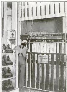
Striking a workman's head, the fender bar automatically brakes the descending elevator
