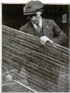
A section of rigid metal lath nailed to studding as reinforcement for plaster or stucco is effective fireproof construction of walls or ceilings
