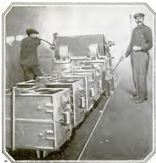
As the cylindrical tank is rotated, molten iron pours from nozzles into molds; two men handle it easily
