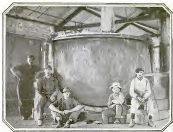
A big caldron raised from the heating well by means of jacks placed under the lifting lugs attached to the rim
