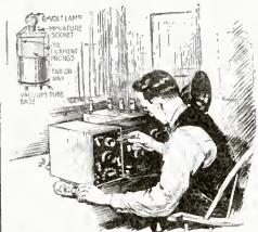
Testing circuits with flashlight bulb
