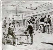
The first telephone exchange, 1855—from a contemporary drawing. Here an operator, seated at a "central" desk, shouted incoming calls to boy assistants who dashed about the room pushing brass pegs into holes and so making connections
