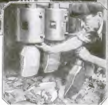
In crushing a cement road, a battery of heavy plungers, with removable chisel-shaped points, shown at right, are raised and lowered by eccentric levers on a shaft driven by the truck motor
