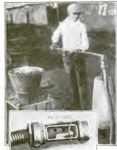
Dropped into the compressed-air tube, the hot rivet opens the valve
