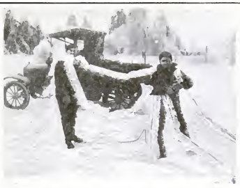
When wires break under tremendous loads of ice, as shown above, marvelous instruments in the central telephone exchange instantly locate the points of trouble along the line, directing an army of repair men in their work of quickly reestablishing communication. Usually the tangled and broken wire is practically worthless
