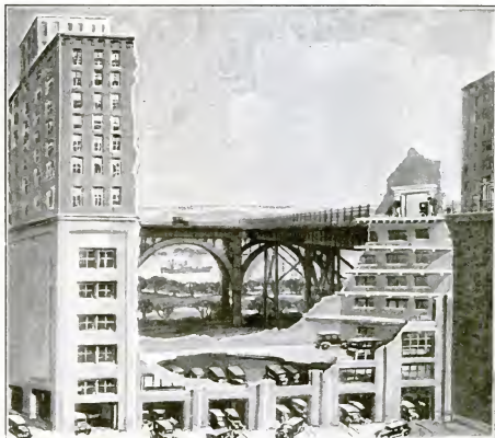
Cutaway view of proposed apartment house showing garages in foundation
