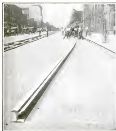
Seven rails, welded together into one, are laid at one time
