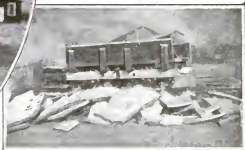
The remains. Fragments of the shattered retort, confined within a 25-foot radius, are easily loaded on cars.
