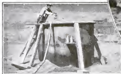
Setting the charge. Into the seven-ton retort, filled with water, are dropped six small charges of explosive gelatin.
