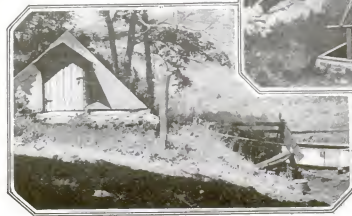
The water from the well above is automatically pumped to two farms. The pump is enclosed in the house to the left. When any faucet is turned on the water works against the piston of the pump
