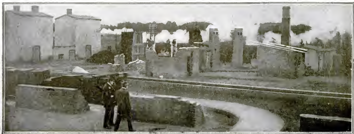
This shows a place where incendiarism is legitimately practised by the proper authorities for the purpose of testing the resistance which iron, steel, stone, brick, cement, and other building materials have to fire
