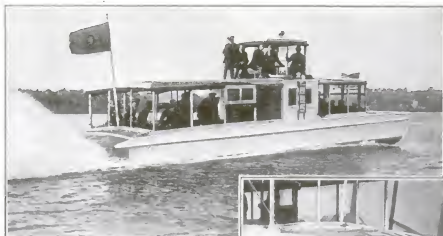
Carrying a load of 51 passengers, this novel sea sled designed for shallow water transportation, recently skimmed over the Connecticut River at a speed of 30 miles an hour
