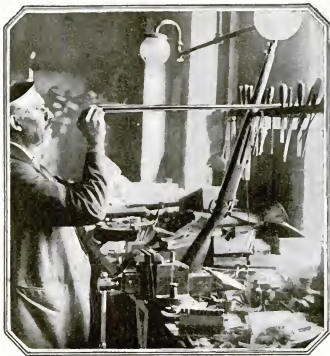
The shop may seem to you to be a hopeless clutter of confusion. It is not. The fact is, Mr. Pope hasn't room for all the lathes and punches and dies and other tools necessary in his business of making rifle-barrels
