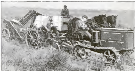
A conveyor carries the potatoes into a wagon moving alongside the machine.
