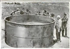
Through the fire unscathed. Here is the tank as it appeared at the conclusion of the test, its contents untouched by the flames
