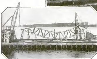
The 150-foot timber cradle used in submerging pipe across three Virginia rivers
