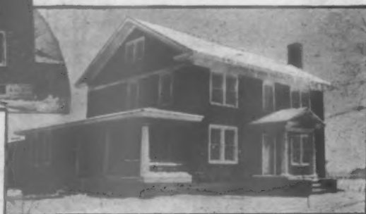
The shingles were dipped in creosote stain before they were put on
