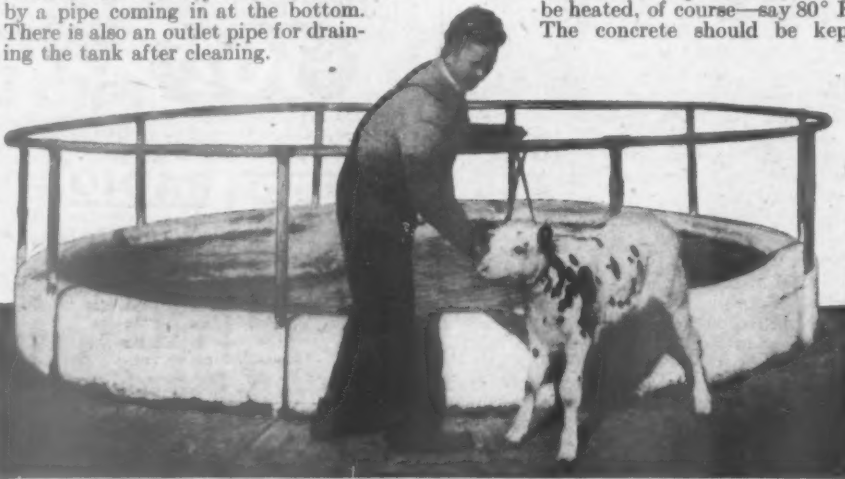
An iron rail keeps the cows from wading in this concrete water-tank
