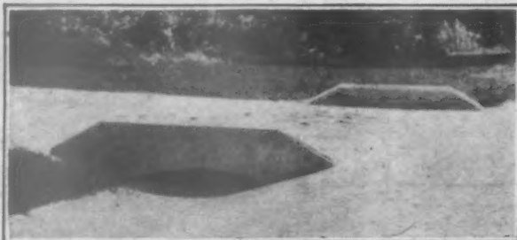
Concrete culvert in a Nebraska barnyard
