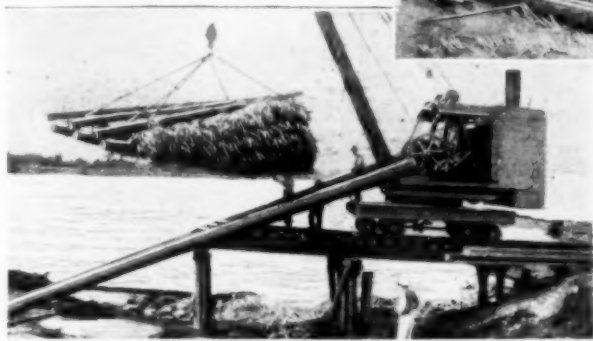
Building the Dam: The Bales of Arrow Weed are Picked Up by Tackle and Run Out over the River on a Cable
