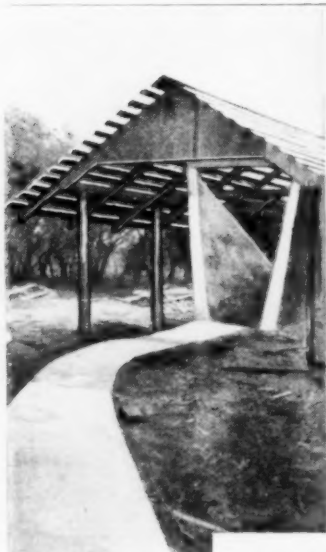
The Concrete Dipping Vat Itself, with the Inclined Entrance Way Visible at the Distant End
