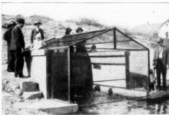
One of the Several Large Springs That Flow into Comanche Creek, and Supply All the Water for the Fort Stockton Project, Protected from Interference by Concrete and Steel
