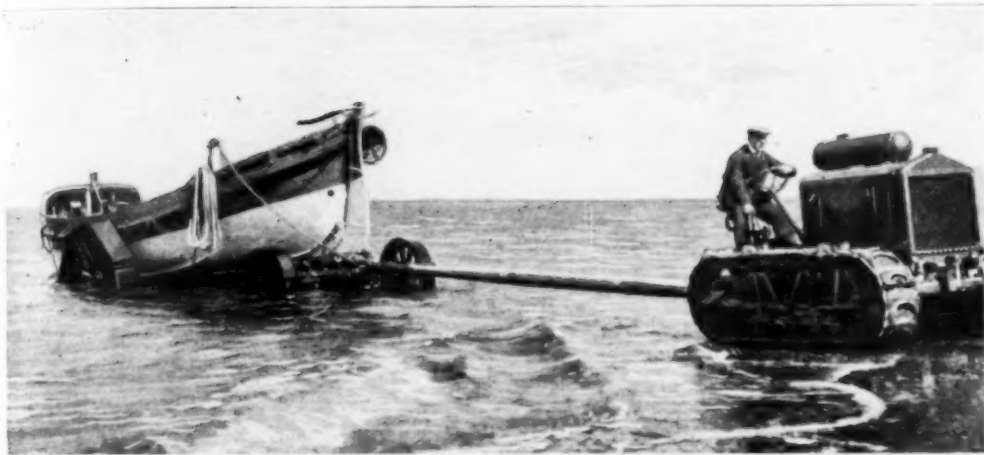
A Lifeboat That is Run into and Out of the Water at an English Seaside Resort, by Means of a Tractor: A Rigid 40-Foot Spar Connects the Tractor with the Wheeled Cradle of the Boat So That Pushing and Pulling Are Equally Effective
