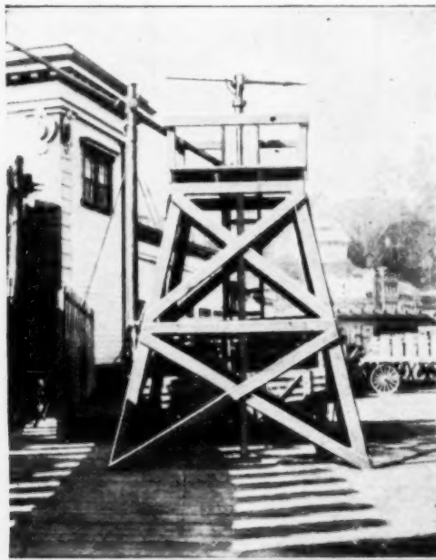
The Swiveling Nozzle on the Top of This Movable Fire-Fighting Tower is Connected to Any of the Fire Hydrants with Which the Docks are Equipped. The Nozzle is Swung Easily in Any Direction
