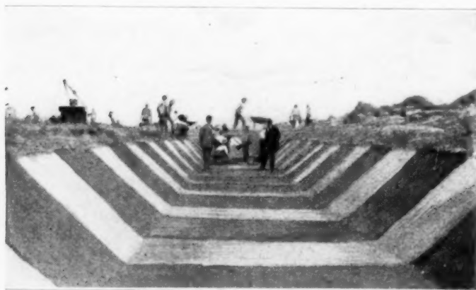
A Concrete-Lined Canal of the Fort Stockton Project under Construction, Leading from the Creek Bed to the Land under Irrigation, with Many Turn-Out Gates and Side Canals
