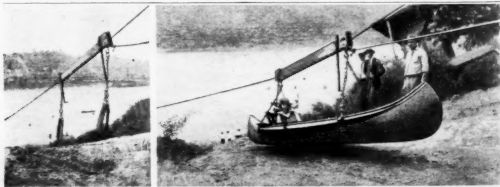
The Cableway Links the Public Boathouse on the Top of the Bank with the Surface of the River, Many Feet Below. Often a Customer Descends to the Water in the Boat He has Rented, as Pictured at the Right. At the Left is Shown the Two Stirrups Which are Placed around the Hull
