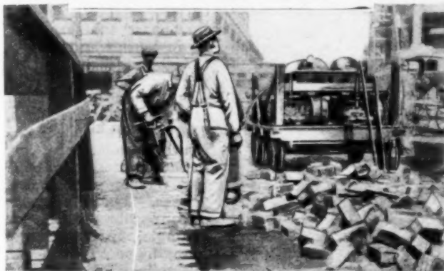
Left: The Motor-Driven Air Compressor, Operating Drills That Cut Holes in the Concrete Base of the Pavement. Right: The One-Ton Iron Ball Dropped onto the Concrete by the Motor Shovel to Break It. This is Used Only When the Pavement Proves Too Hard for the Drills to Penetrate
