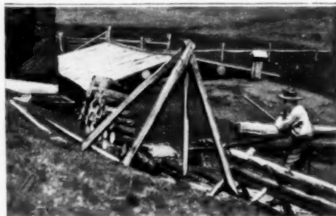
By Pivoting One End of His Tool to the Pendulum-like Scantling, the Forest Ranger is Enabled to Use the Two-Handed Saw
