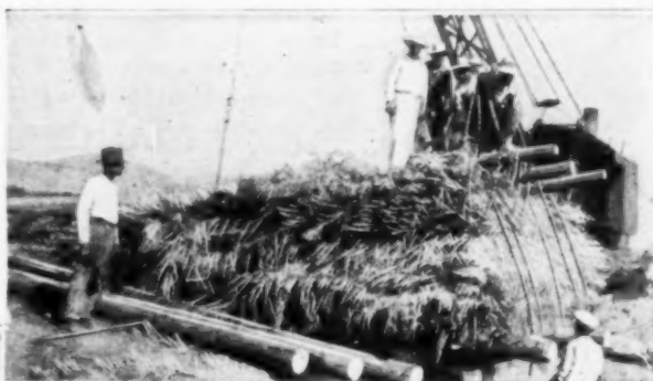
Making Bales of Arrow Weed, Cut from the River Itself, to be Used in Building the Peculiar Dam
