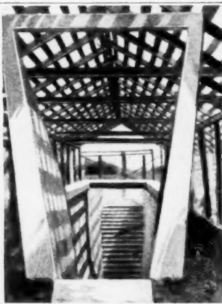
Looking across the Vat at the Exit Stairs That Take the Place of the Usual Unsafe Incline
