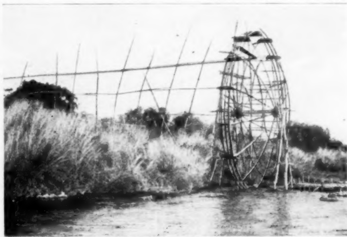
This Water Wheel, Reminiscent of the Type Used in the Historic Valley of the Euphrates, Elevates Water to the Bamboo Trough, Whence It Flows to the Fields of a Philippine Farm. This Primitive System Works Satisfactorily
