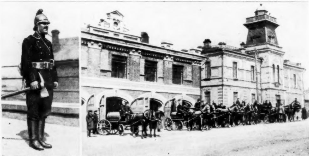
A Siberian Fire Fighter of Vladivostok, and the Station and Equipment of the City Fire Department: The "Engines" Are Merely Tank Wagons, from Which the Water is Drawn by Means of a Small Hand Pump
