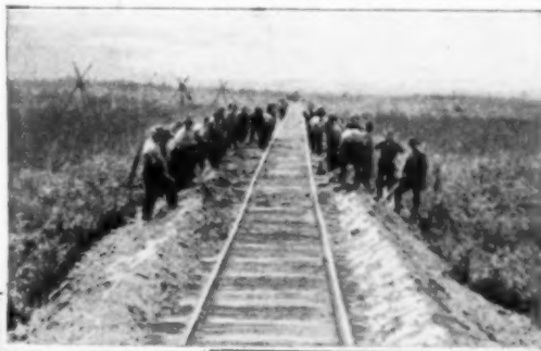
Laying Track across the Tundras: The Ballast is Laid on Logs Sunk in the Swamp
