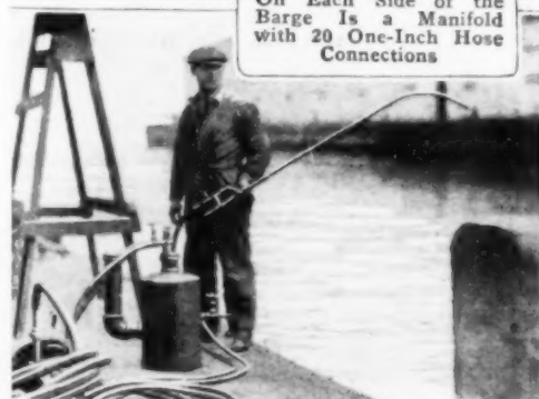
Sand Dropped into These Tanks from the Hoppers is Expelled at High Velocity
