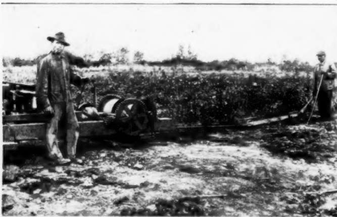
The Stationary Engine and Winding Drum at the Left Pull the Plow at the Right with a Cable, and the U-Shaped Blade Cuts under the Roots of Small Trees and Lifts Them from the Ground
