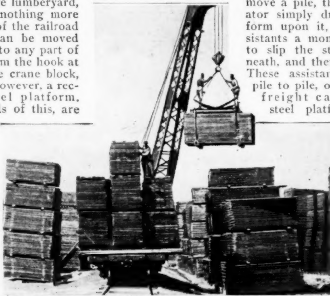
One of the Standardized Piles of Lumber is being Loaded upon the Freight Car in the Foreground by the Stacking Machine. This Is Simply a Railroad Crane from Which is Suspended a Rectangular Platform with Two Stirrups of Chain
