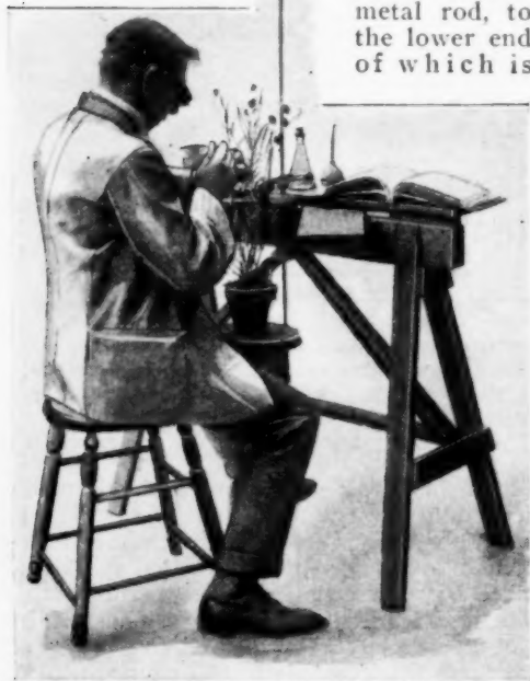
Owing to the Difficulty of Bringing the Blossoms of a Plant to the Proper Elevation, a Plant Hybridizer Evolved This Adjustable Table
