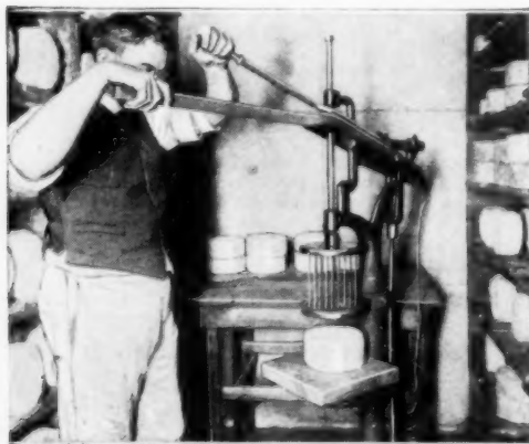
This Machine Riddles the Cheese with Many Holes and So Hastens the Growth of the Mold, or Fungus
