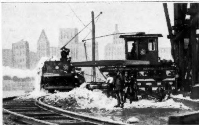
The Battering Ram Carried by the Car at the Right Pushes the Load off the Flat Car and into the River
