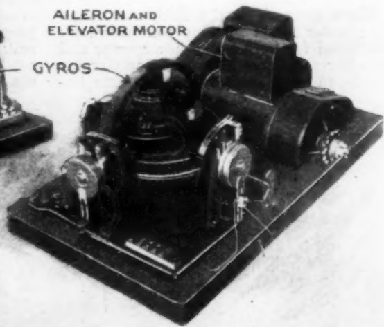
This Is the Unit Seen, at the Top of the Page, Just in Rear of the Pilots' Seats. It Preserves Lateral and Longitudinal Stability in the Same Way That the Other Unit Maintains Direction
