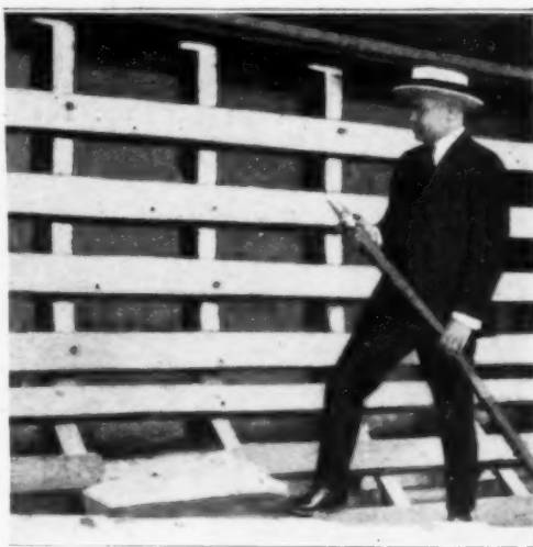
Using the Sand Blast, the Workmen can Clean the Plates of the Hold without Removing the Protecting Timbers
