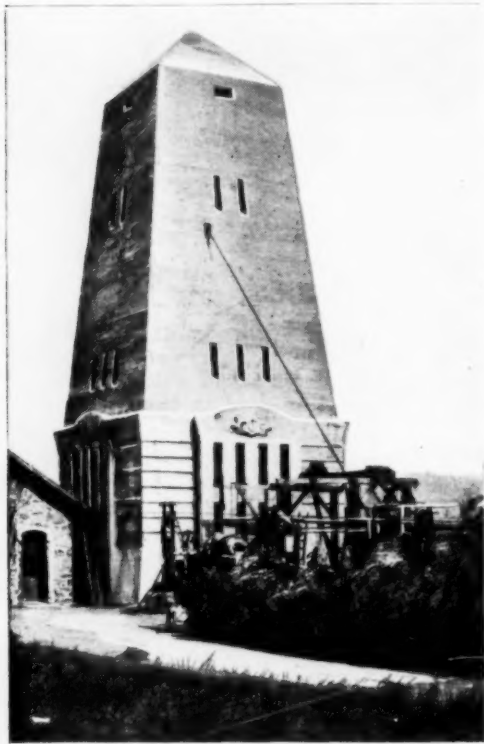
This Concrete Obelisk Is Not a Monument, but a "Headframe" over the Mouth of a Michigan Iron Mine
