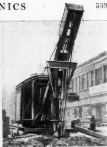
The Big Motor-Driven Shovel Operated by Trolley Current, Used to Tear Up the Pavement or to Crack It by Dropping a Weight
