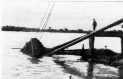
Left: Sinking the Bale in the River, by Attaching It to a Cable and Allowing the Current to Carry It to the Bottom. Right: The Nearly Completed Dam of Arrow Weed, Holding Back the Swift Colorado River
