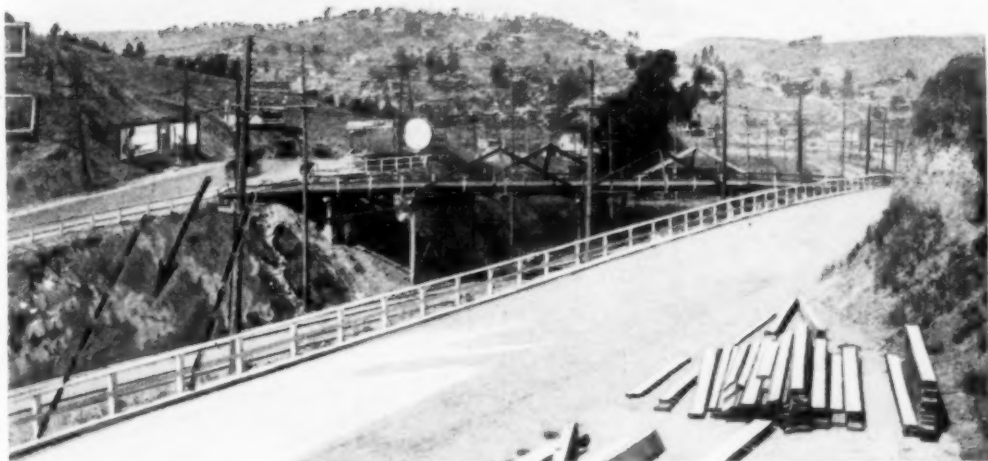
Across the Old Bridge, the Location of Which is Indicated at the Left, Motorists could Pass from One Road to the Other with Speed Unabated. Many Fatal Accidents were Attributed to This Condition. The Bridge was Rebuilt in the New Position, Recently, to Make This Speeding Impossible
