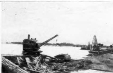
Left: Sinking the Bale in the River, by Attaching It to a Cable and Allowing the Current to Carry It to the Bottom. Right: The Nearly Completed Dam of Arrow Weed, Holding Back the Swift Colorado River
