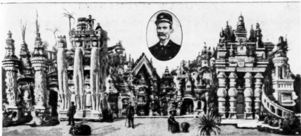
Five Different Types of Architecture Appear in the 85-Foot Façade of the Extraordinary Palace, Inspired by Oriental Pictures, and Laboriously Constructed by the Poor French Postman Portrayed in the Insert
