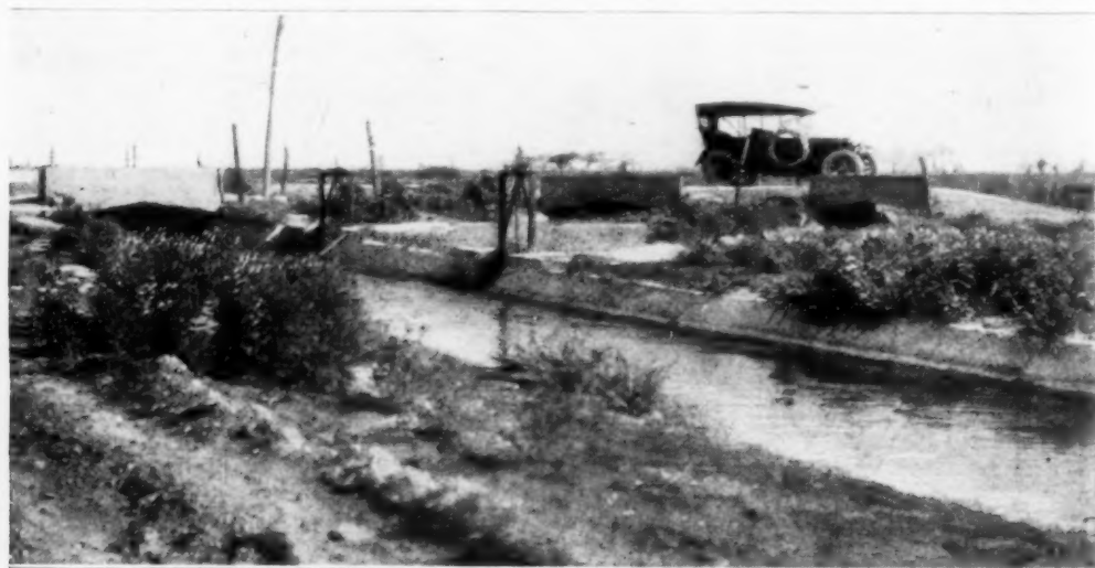
Just This Side of the Bridge, to the Left, are to be Seen Two of the Iron Turn-Out Gates, Set in Concrete, and Capable of being Raised, Lowered, and Locked in Any Position
