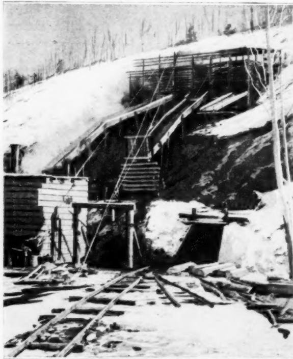
Near "Mile 365" a Coal Mine has been Developed Right at the Side of the Track, Making It Unnecessary to Penetrate the Extensive Coal Fields Themselves. The Lower Opening into This Mine Passes under the Main Line of the Railroad
