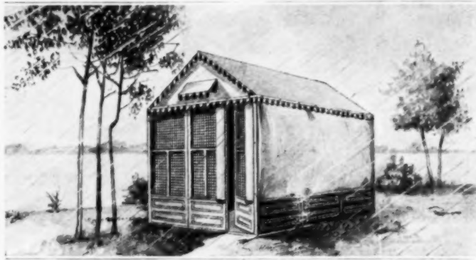
The Storm Curtain has been Withdrawn from the Front Wall of the Lawn Cottage to Show Two of the Screened Panels Which Form the Walls. The Structure can be Erected in an Hour
