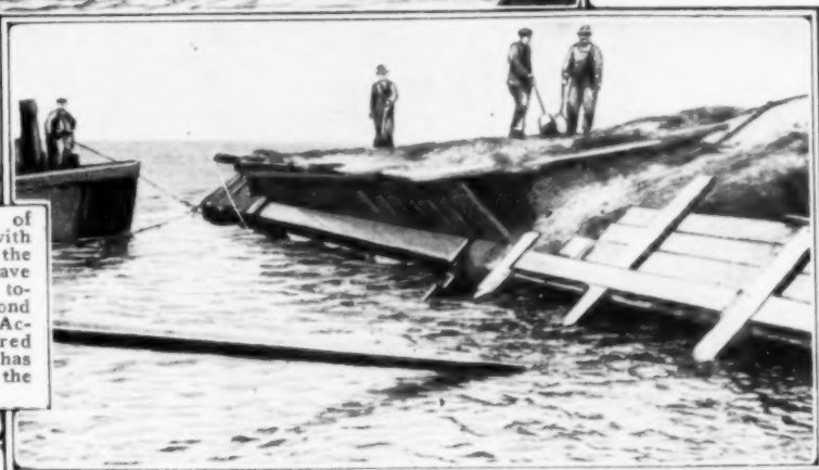
The Unusual Expedient of Piling Gravel on the Exposed Side was Employed Recently to Right a Big Auxiliary Schooner Which had been Overturned by a Tide Rip in Puget Sound. In This Photograph the First Row of Cribs is being Spiked to the Wooden Hull
