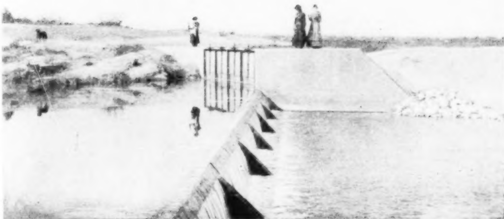
The Concrete Diversion Dam in Comanche Creek That Turns the Waters of the Springs into the Concrete-Lined Canals, and through the Numerous Turn-Out Gates, to Irrigate the Big Fort Stockton District
