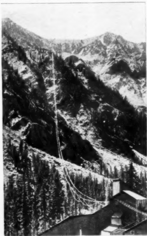
From the Crushing Mill in the Foreground the Cableway is Seen to Stretch Upward for More than a Mile to the Gold Mine on the Summit
