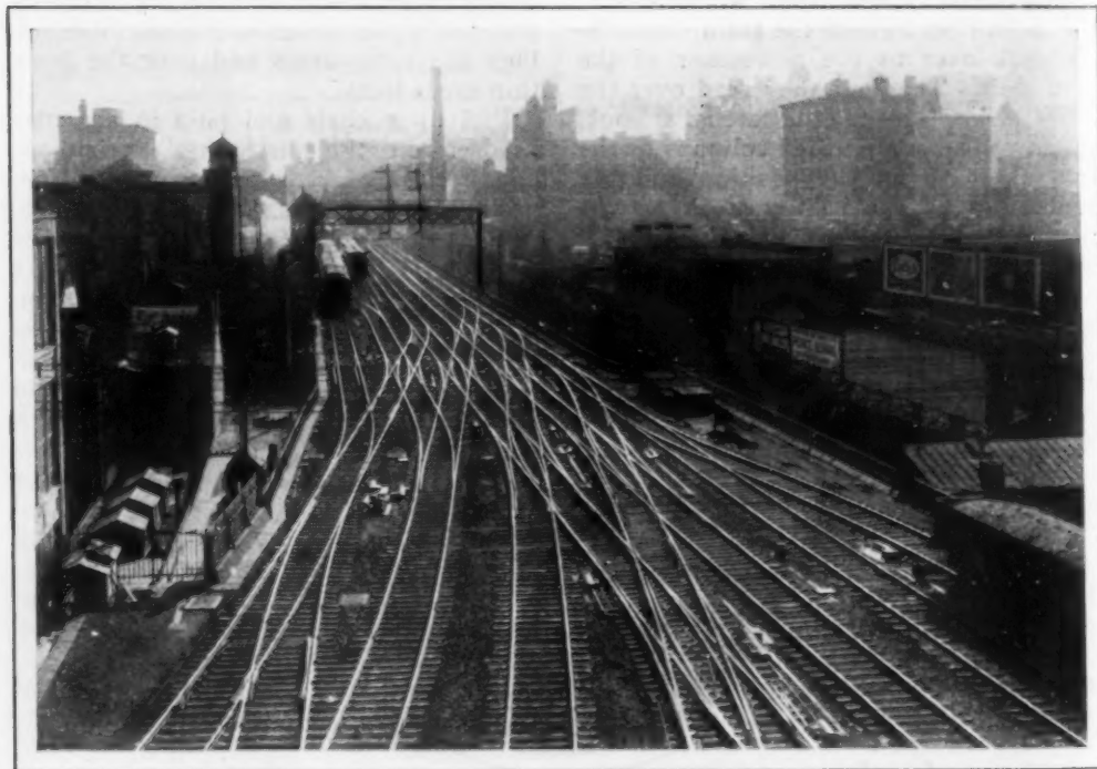
Electric Interlocking Signals Control the Network of Tracks Leading Out of the Terminal and Guide the Trains over the Route Designated by the Dispatcher's Office
