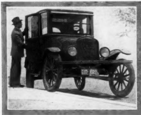
Put One Wheel on the Curb and Try Doors to See If They Bind; Also Inspect the Spark Plugs for the Uneven Formation of Carbon
