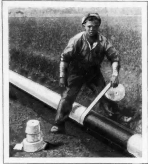
Embalming a Gas Main; This Expert Taper Can Cover a Twenty-Foot Length in Two Minutes
