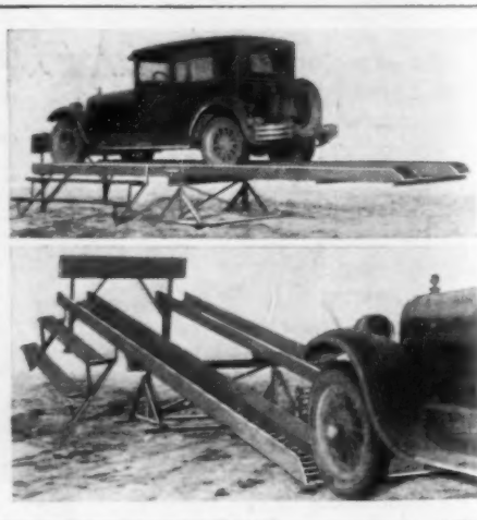
Car in Level Position on Tilting Rack, and About to Ascend; Note Wide Runways for Wheels
