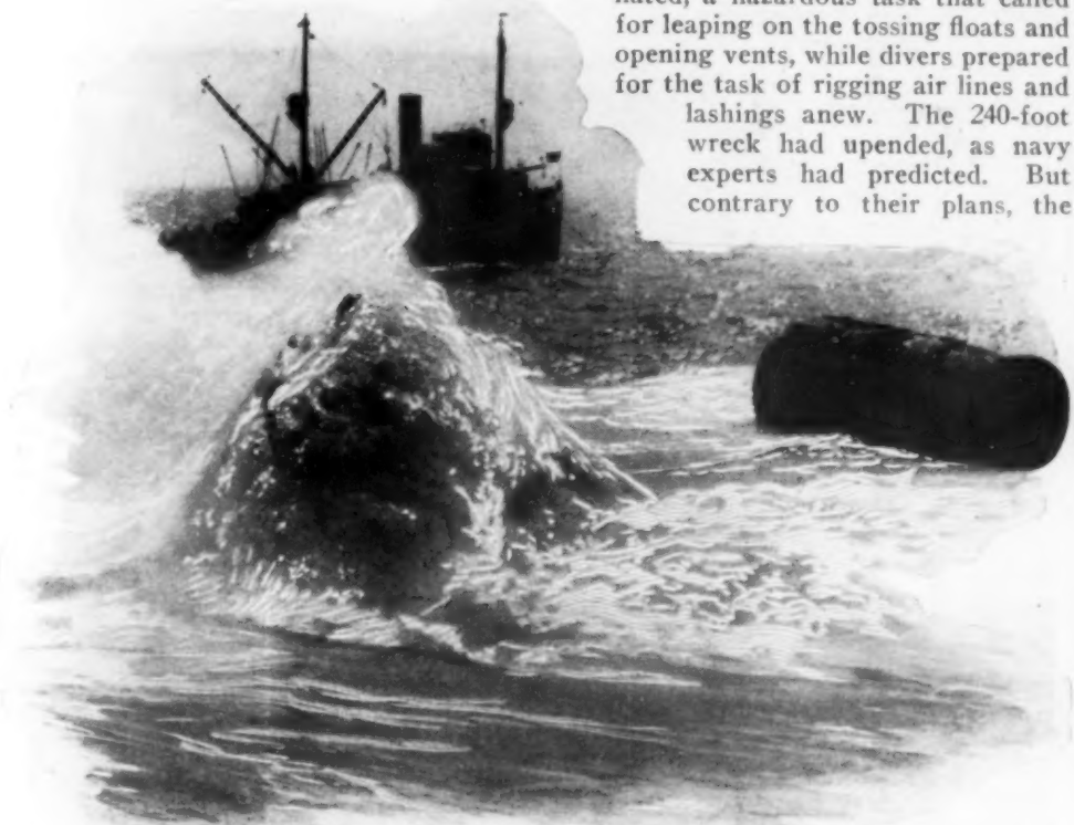
Why the "S-51" Slipped Back after the First Raising; Pontoons Lashed to the Stern Broke Loose and Leaped to the Surface; Photo Shows One Coming Up
