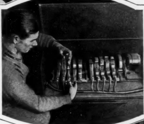
The Making of Electric Signs Is a Highly Skilled Profession; Center Shows a "Flasher" Assembly for an Animated Advertisement
