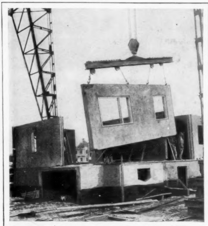
Where Derricks Serve as Masons; Lowering Side of Concrete House as Unit to Foundation during Rapid Construction
