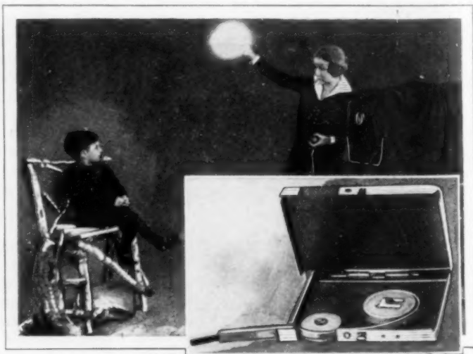
Taking Studio Flashlight with Magnesium Tape and Close View of Igniter Opened, to Show Material Coiled in Position for Use
