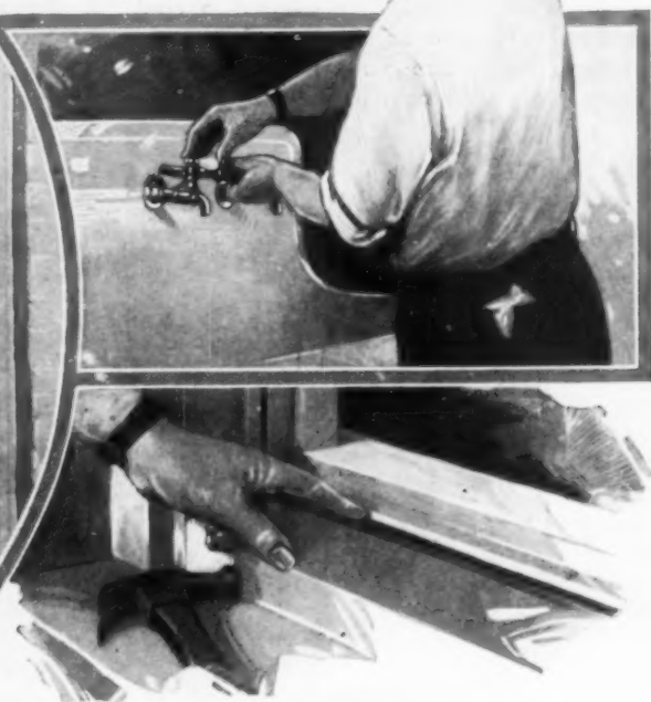
Left, Applying Weather Stripping Is a Simple Method of Saving Heat; Lower Right, an Effective Metal Strip
