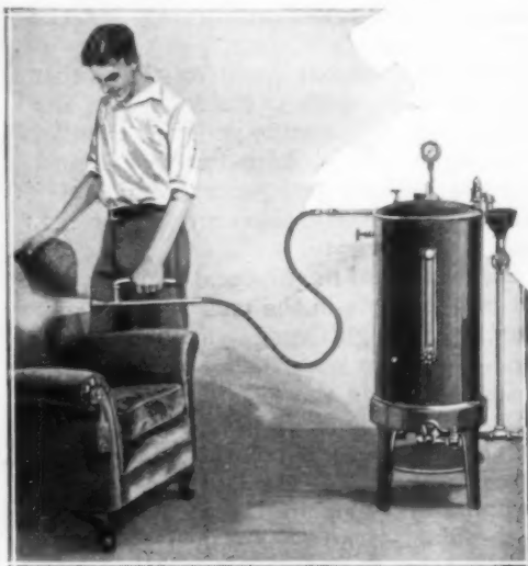
Steam Cleaning an Upholstered Chair with Handy Boiler Outfit; Control Nozzle Regulates Blast
