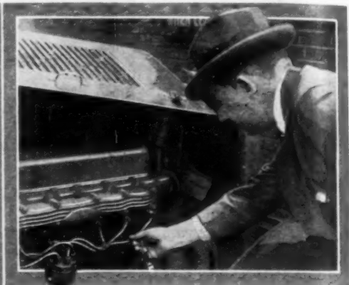
Put One Wheel on the Curb and Try Doors to See If They Bind; Also Inspect the Spark Plugs for the Uneven Formation of Carbon
