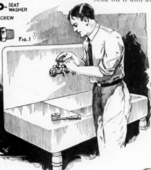
How Common Compression and Fuller Faucets Are Taken Apart for Renewal of Balls and Washers or Redressing the Seat
