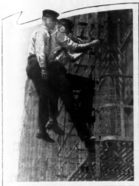
Three Important Uses of the Combination Belt; Rescuing, Taking Hose up Ladder and Steadying Nozzle
